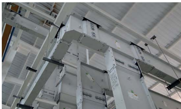
Example of Legrand busbar system
